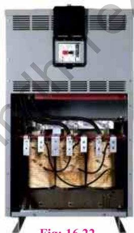
Fig: 16.22 Transformer in high voltage circuit breaker
