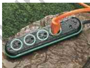
Fig: 15.24 Electrical extension placed damped environment
